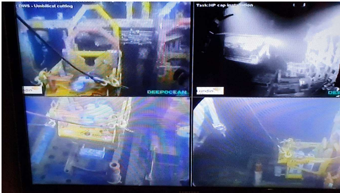
Photo #3 Installation of High Pressure Cap on Pierce RBM (Riser Base Manifold)
