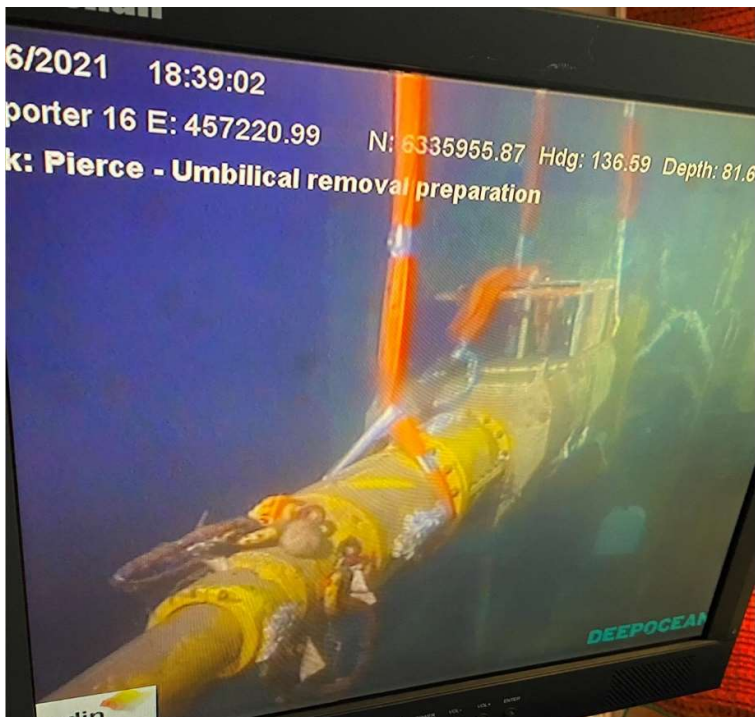
Photo #2 Umbilical disconnect from Pierce RBM (Riser Base Manifold)
