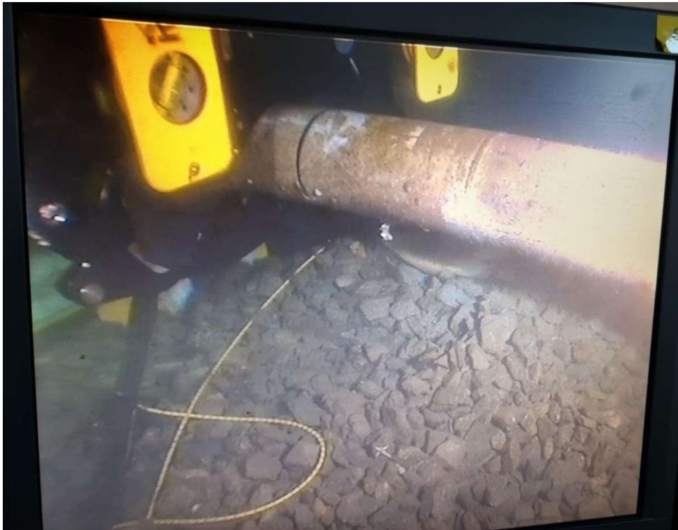
Photo #4 Cutting of production flowline with Diamond Wire Saw
