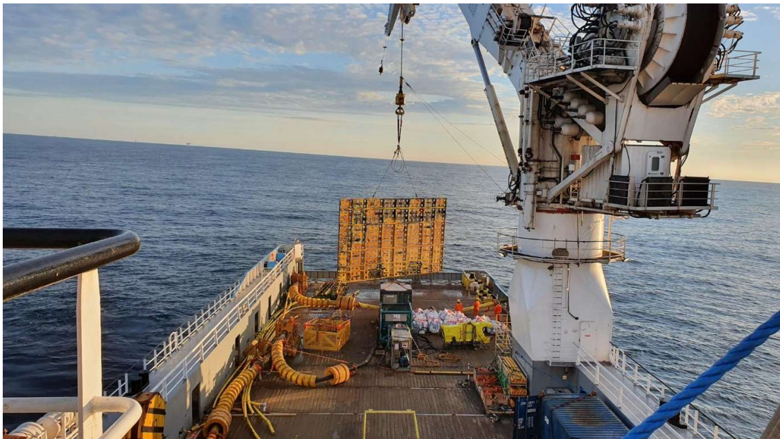
Photo #8 Recovery of PLET support frame
