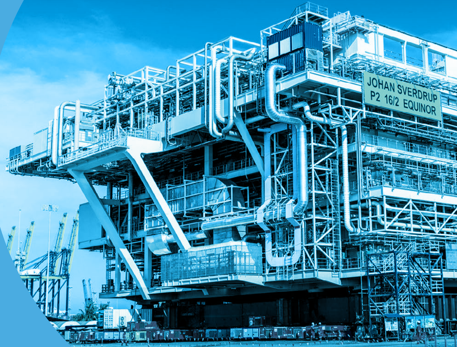
Module support frame sail away - Thailand
