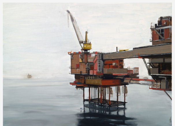
Cutting the legs of Valhall DP. An oil platform under decommissioning process.
