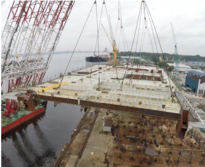
30 January 2015: Lifting of the intermediate deck
