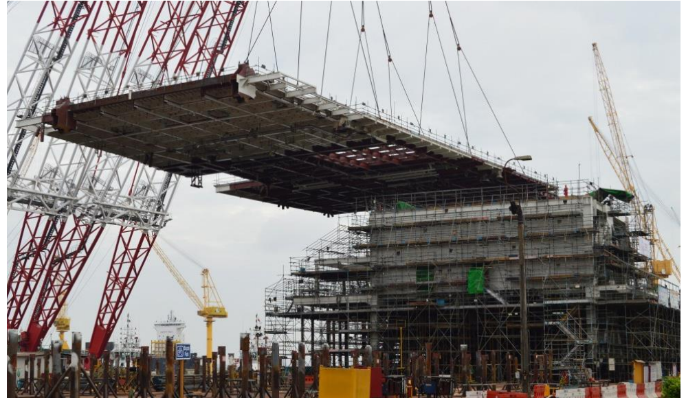
The 3 500 m 2 intermediate deck fit well together with the cellar deck
