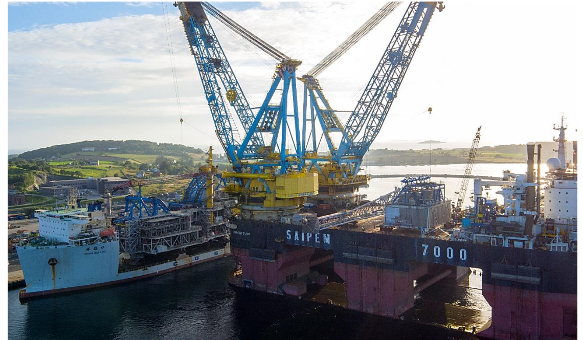
Flare and M50 module lifted onto Saipem 7000
